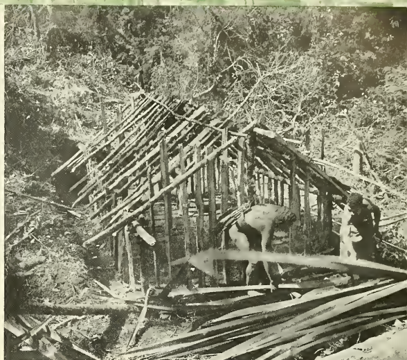
▲ House for cargo boys under construction. Four men can build such a house in two hours. The roof will be nearly a foot thick, and fire will be kept burning day and night, for it is cold at this altitude of 8000 feet. It will shelter a dozen men
