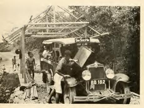
On NIAS, bridges are covered to save the wood from the constant rain. This bridge, in course of construction, will look much like an old-fashioned New England covered bridge when it is finished. The open hood of the automobile and the towrope on the bumper suggest that travel in Nias has its difficulties
