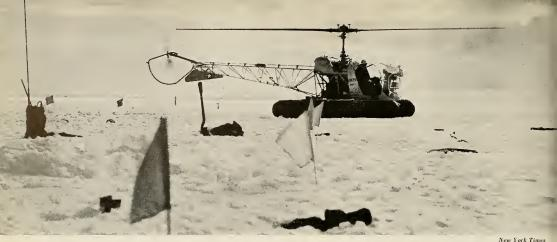
A "WHITE-OUT" is the greatest danger encountered by pilots in the antarctic. When there is no sun to bring the snow surface into focus, pieces of wood are dropped as markers. The helicopter in this picture, equipped with pontoons, is still on the ground although it looks as though it is hovering above.
