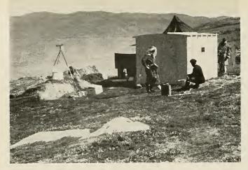
PORTABLE LABORATORY, built of prefabricated plywood panels, was twelve feet long, eight wide. Designed for seven people, it frequently held eight.
