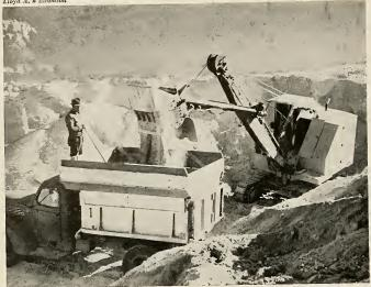
A A STEAM SHOVEL loading a truck with pumice. The material is so light that the bucket was enlarged by 65%.
