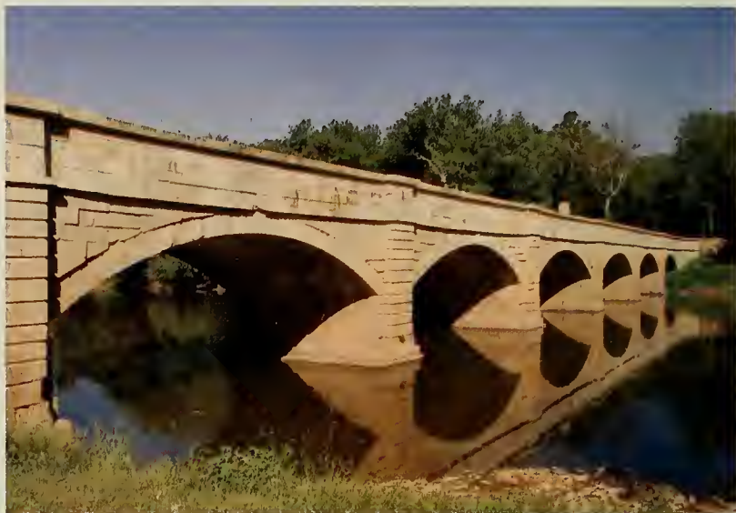
The 438-foot Monocacy Aqueduct is the largest aqueduct on the Chesapeake and Ohio Canal, crossing the Monocacy River just before it empties into the Potomac River.
