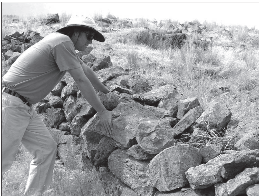
FIG. 3. Rubble-fill construction pattern of the Fort Sage Drift Fence.
