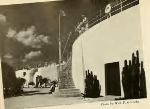
(Left) THE CONCRETE SHELL surrounding the steel tanks encloses observation corridors. Stairways lead to a top deck from which the surface of the tanks can be viewed. Flocks of pelicans pass overhead continually and egrets dot the marsh expanses to the west
