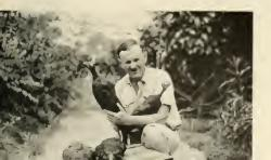
Doing his but for the "gold standard": a Somiba workman in the placer mine at Augumu agitating goldbearing gravel to separate the heavier precious metal
