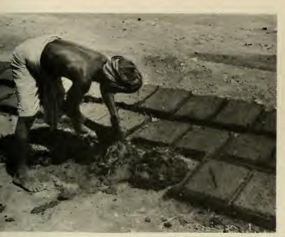
(Above) SUN-DRIED BRICK is the universal building material. The clay is mixed with water and cut straw according to the ancient formula
