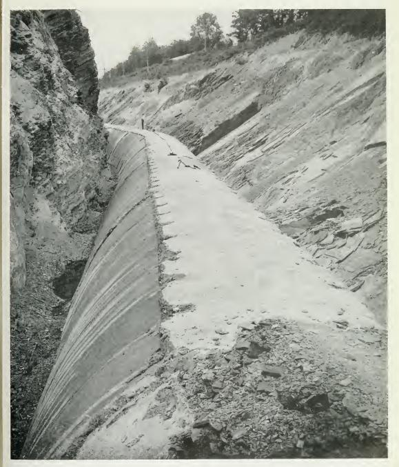
THE CONCRETE CONDUIT SEVENTEEN FEET INSIDE MEASUREMENT
