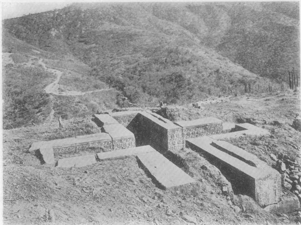
CRUCIFORM CHAMBER. LOOKING SOUTHEAST, BEFORE EXCAVATION. UPPER GUAROO.
