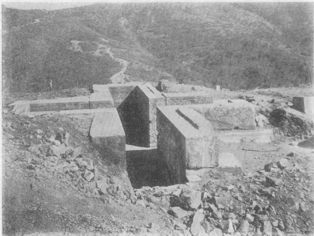
CRUCIFORM CHAMBER. LOOKING EAST, AFTER EXCAVATION. UPPER GUIAROO.
